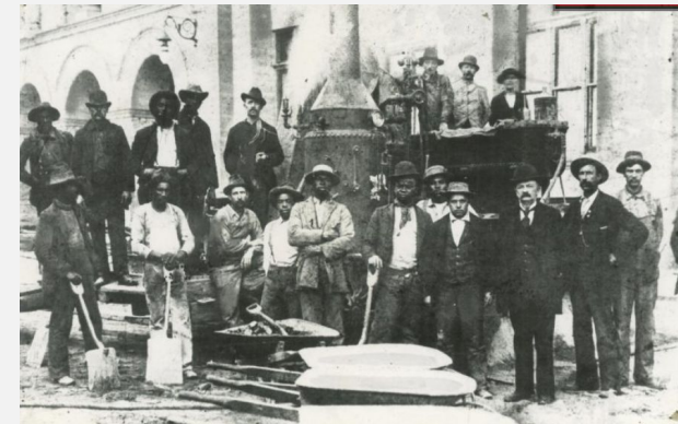
Construction Workers at Milwaukee City Hall, 1896 The Encyclopedia of Milwaukee
